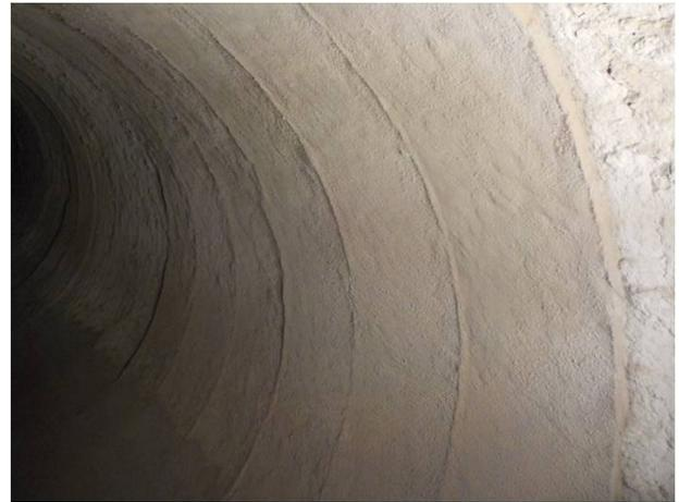
**Fig. 3:** Aspect of the ALFRAN castable installed.
